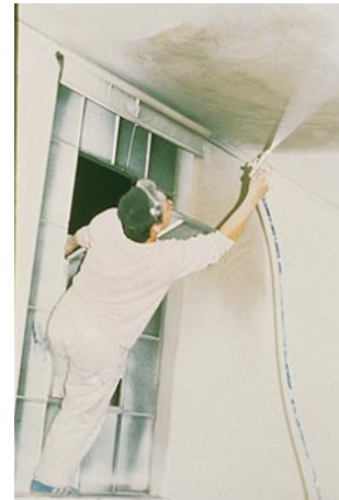
Cheryl Swannack spray painting ceiling during construction of the new space on Spring Street. (Photo from the Woman's Building Image Bank.)
